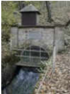
Opening of a mine tunnel [2]
