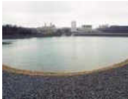
Water treatment plant Königstein [3]
