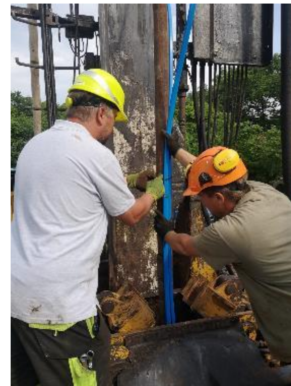
During multipacker installation
