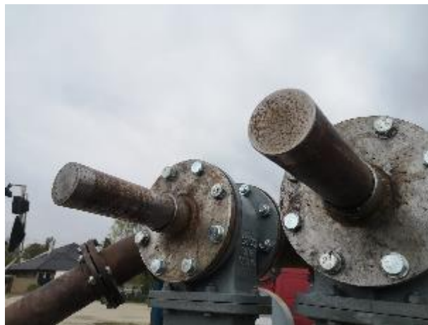
High p / High T probes on the wellhead
