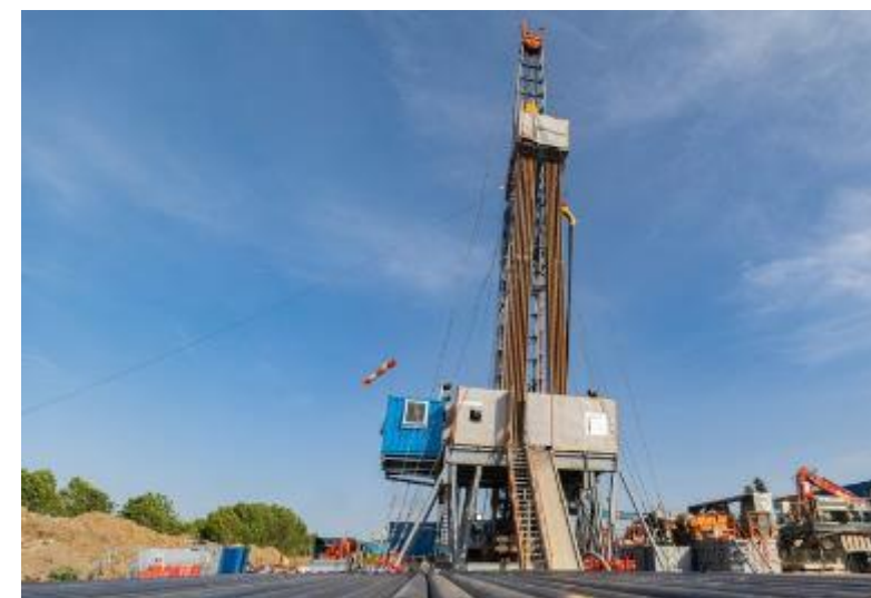
Drilling rig, during geothermal drilling
